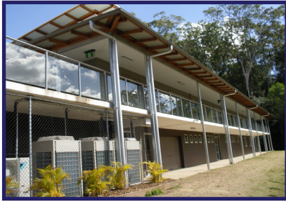
Sunshine Coast Grammar School Structural, building hydraulic and civil design and supervision of Sports Performance Centre.
