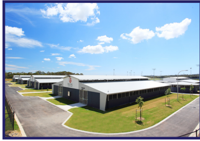
Stabling Complex, Corbould Park Racecourse Structural, civil & hydraulic building design and project management of major stabling complex (416 No.) & associated facilities.
