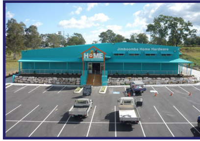
Home Hardware, Jimboomba Structural, civil & hydraulic design, project management, project specifications, tender analysis, and superintendent services.
